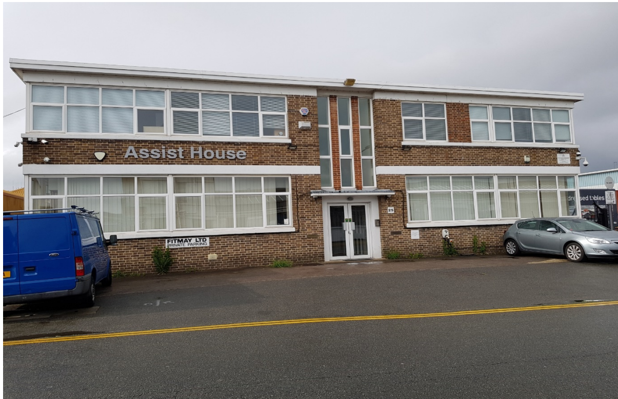
Assist House, 25 Lombard Road. (Fitmay House)
